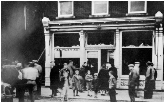
Waveland citizens survey the damage to the bank's exterior
