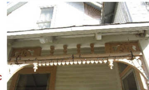
ABOVE: 'GINGERBREAD' TRIM TYPICAL OF VICTORIAN ERA INDIANA CONSTRUCTION
